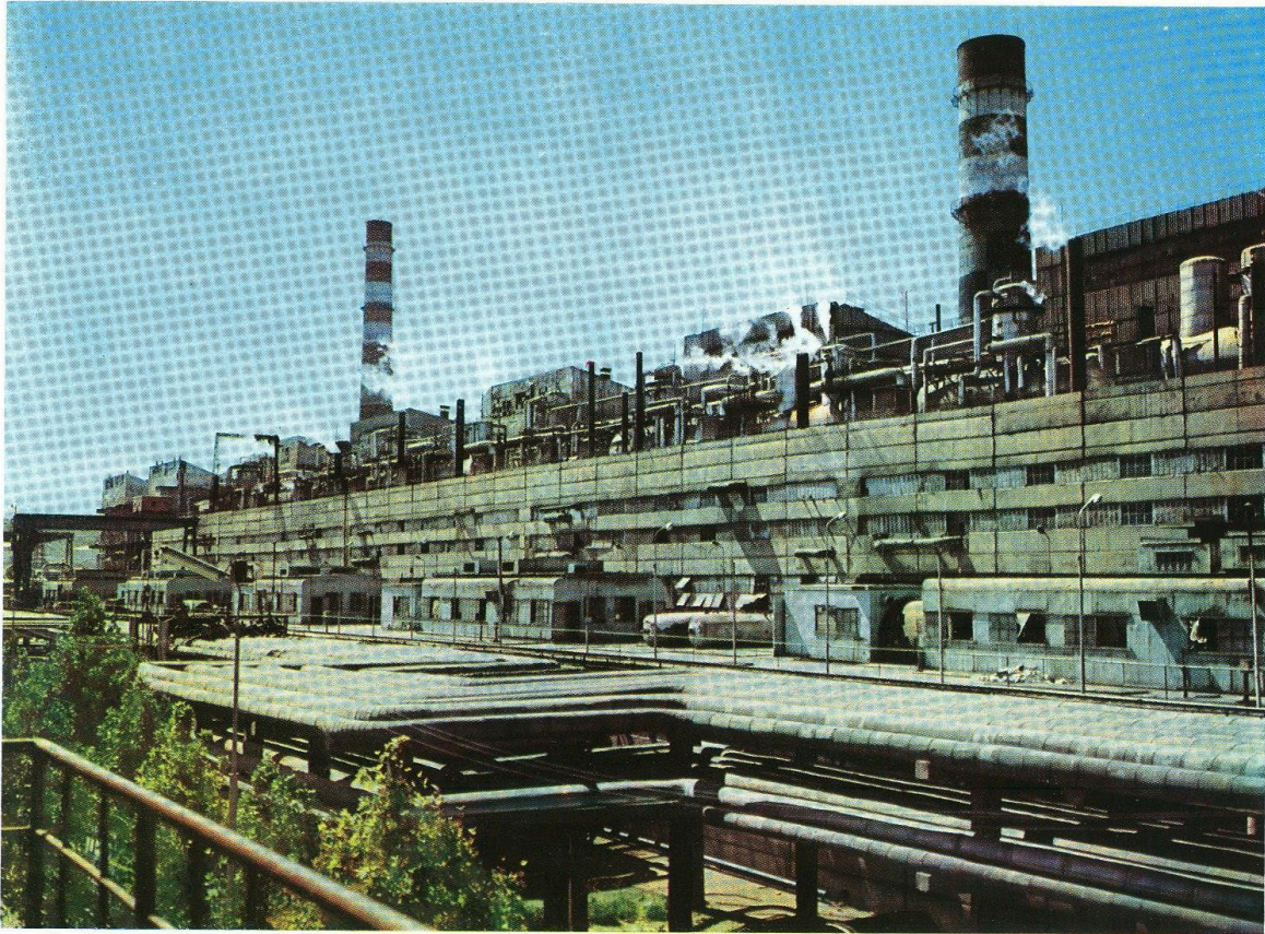
Yerevan Heat-Electric Generating Plant. General View
