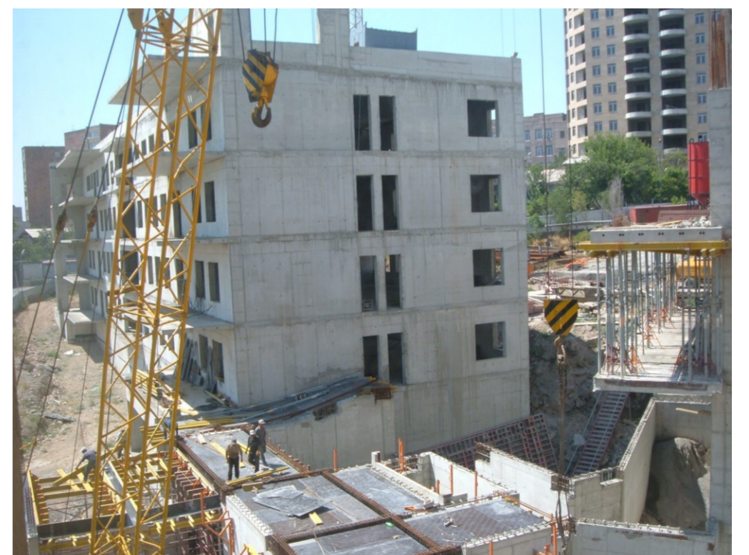
The Avedisian building in progress
