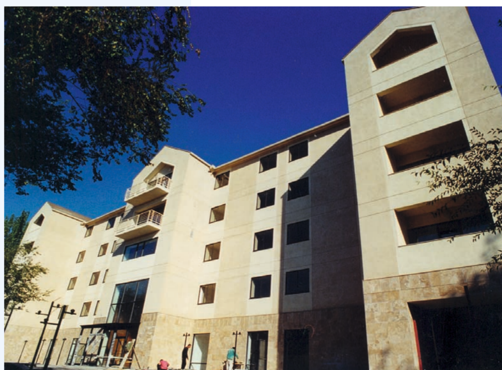
The completed AUA Center on Alex Manoogian Street
