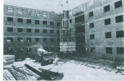
"AUA Center under construction"
