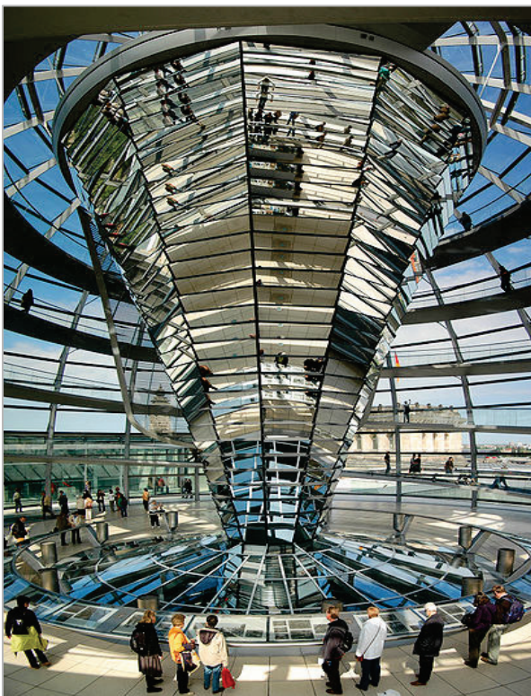
Figure 8. Interior view of the glass dome of the Reichstag in Berlin, Germany, by architect Norman Foster, another iconic masterpiece of daylighting. The dome also allows for natural ventilation from the top of the dome, similar to the Pantheon in Rome
